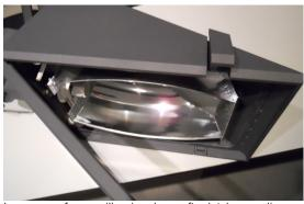
Lens cover frame will swing down after latches unclip
